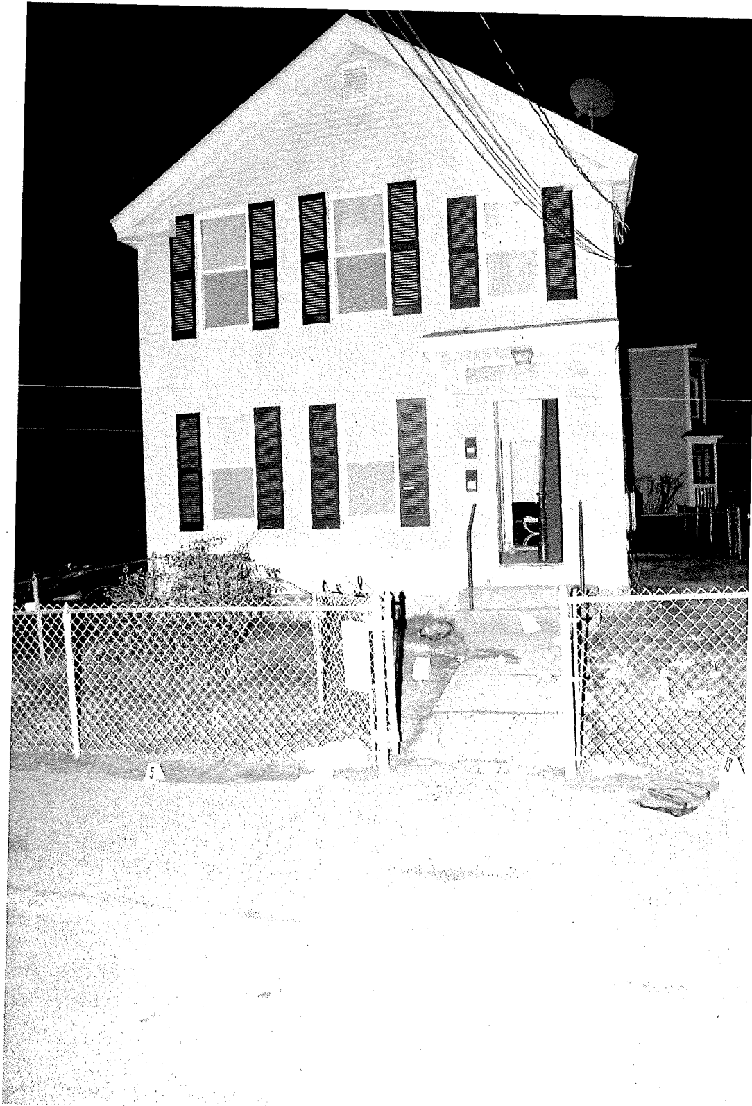
View of the front of 75 Cambridge Street from the street
